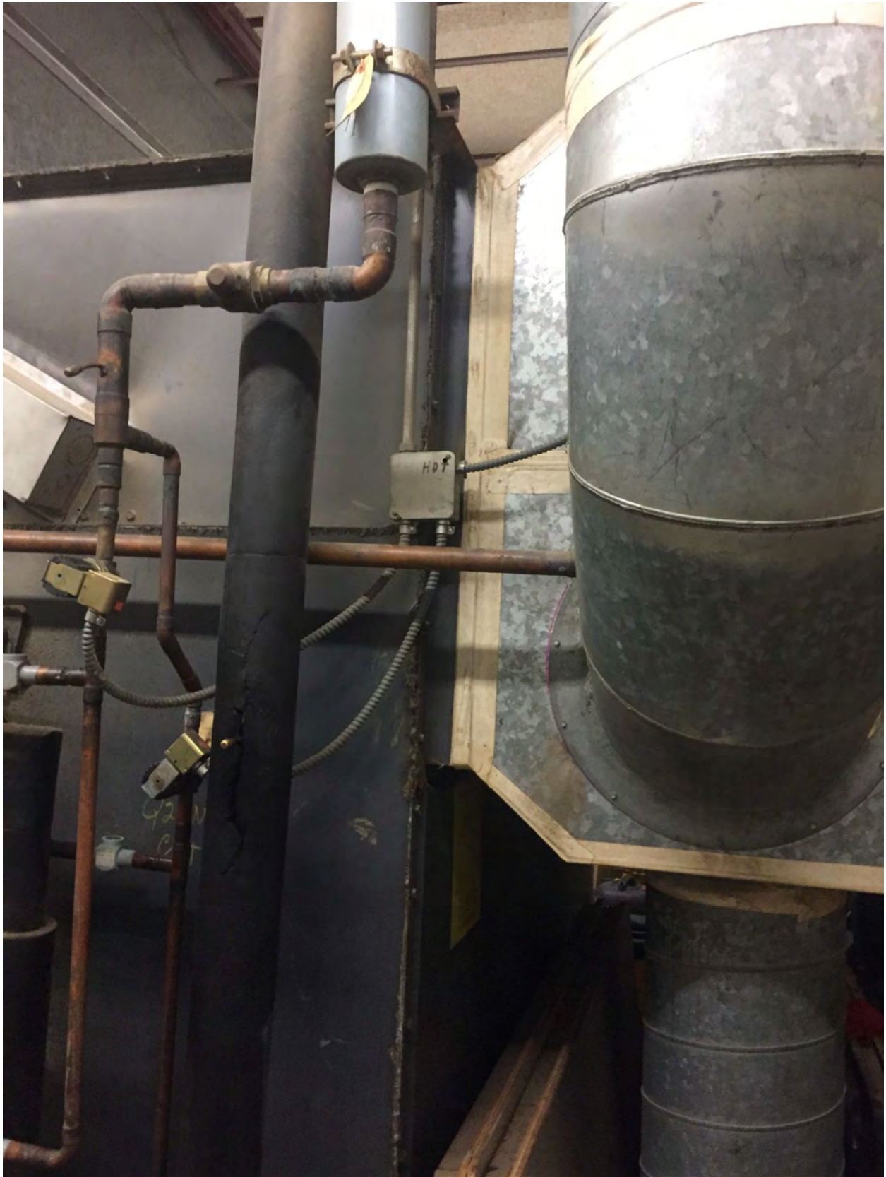
Supply air connection
