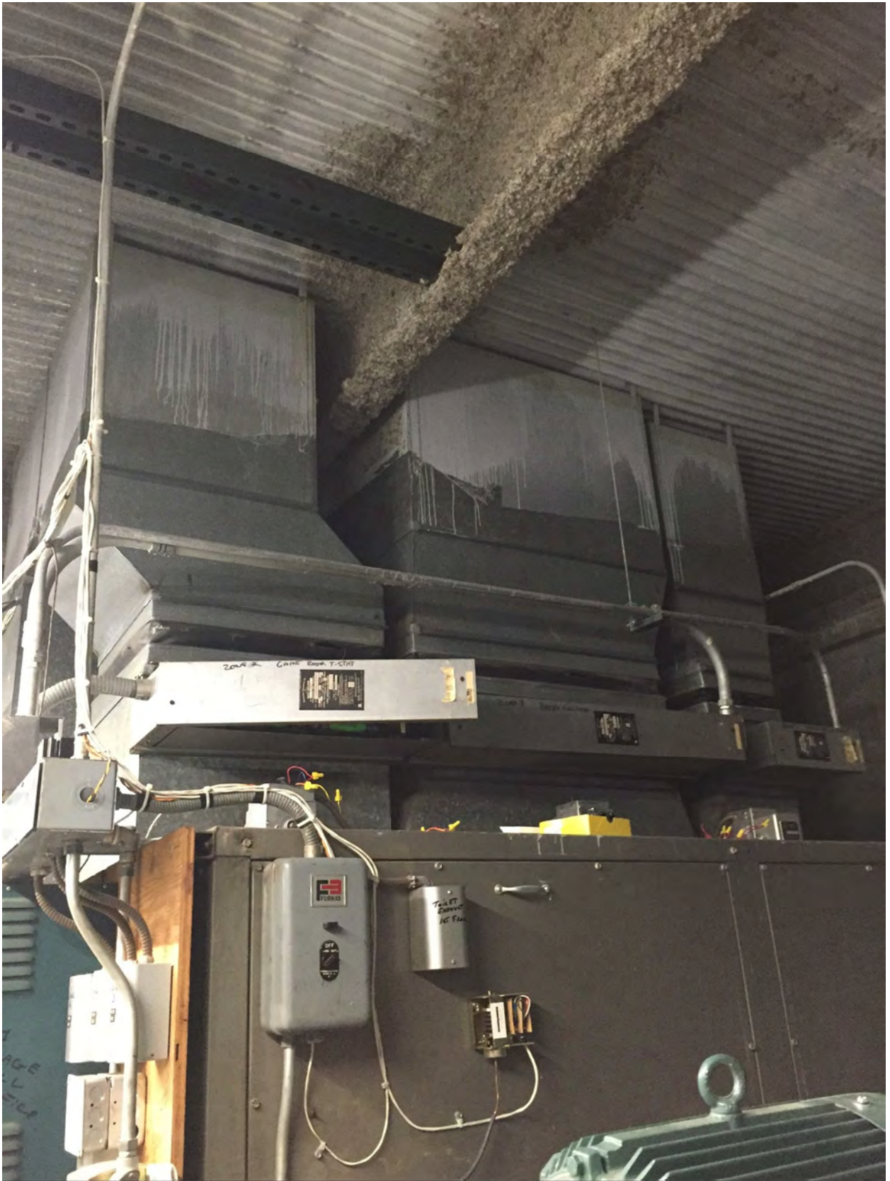
Supply air connection
