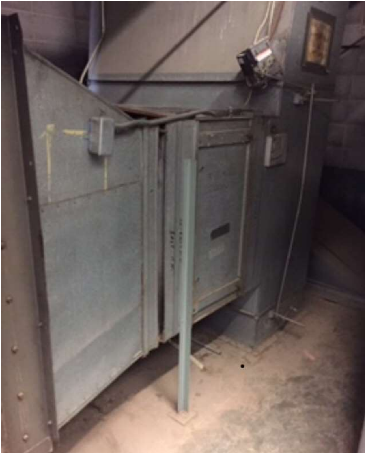
Return and outside air connection
