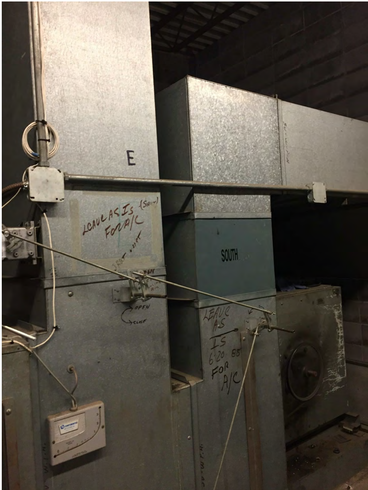
Return and outside air connection
