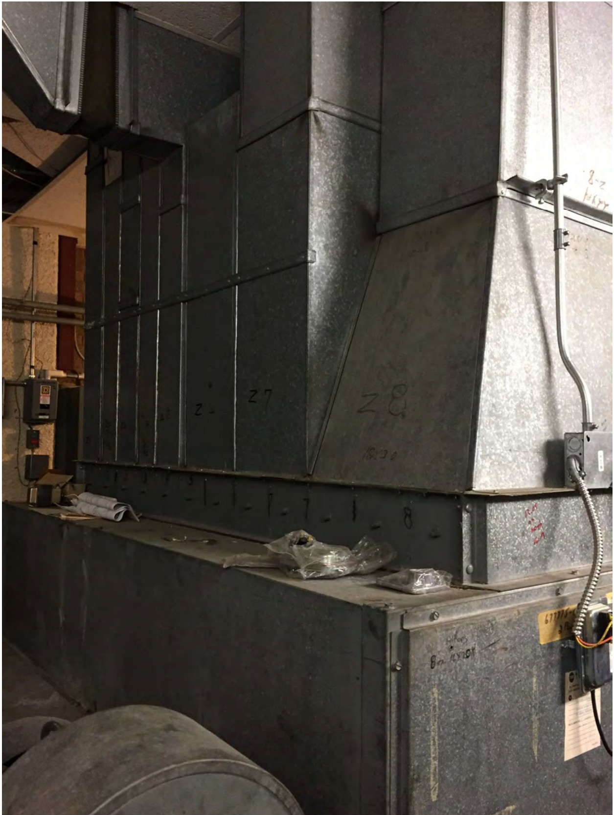
Supply air connection
