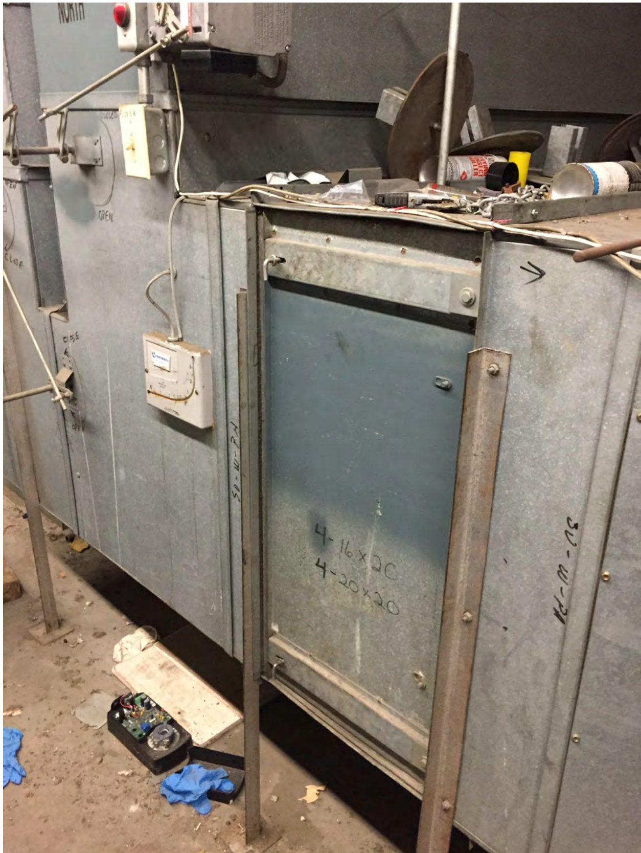
Return and outside air connection
