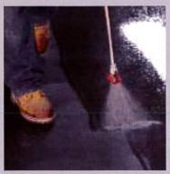
DRYCRETE CURE SHIELD is applied at a coverage rate of 150-200 Sq. Ft. per gallon on broom finished surfaces and 200-300 Sq. Ft. per gallon on hard troweled floors.
