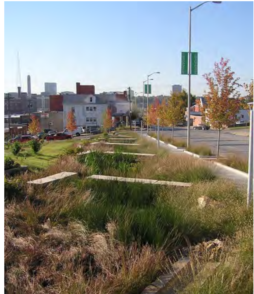
Example of Vegetated Swale and Ledgerock Weirs (18th & Broadway, Kansas City)
