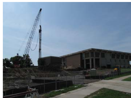
Construction of Remington Hall is underway.
